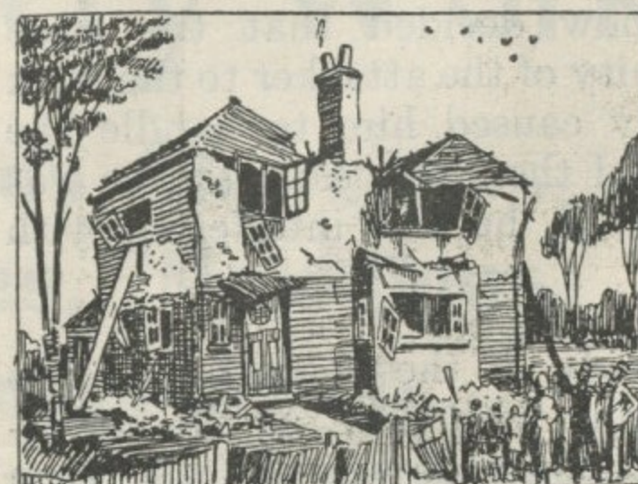
In a Jerry-built House
