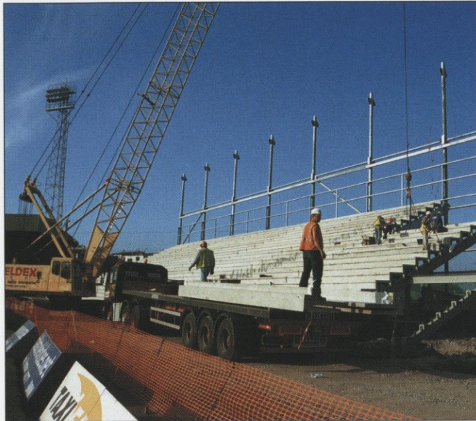
The concrete steps are lowered into position
