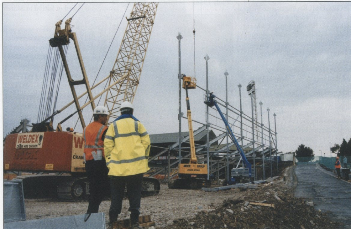
Mechanical means to set up the frame work.
