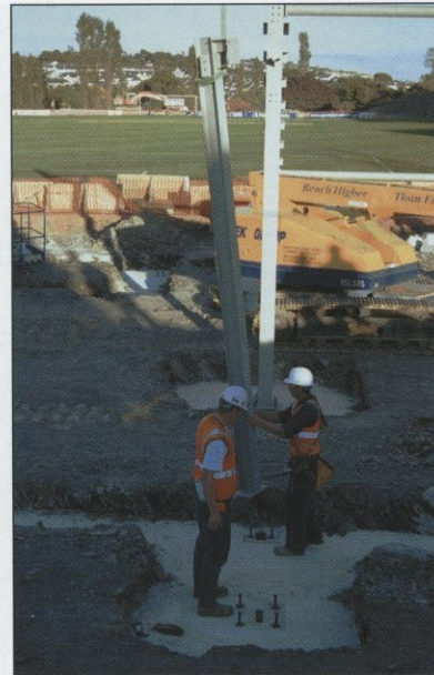
The positioning of the uprights.
