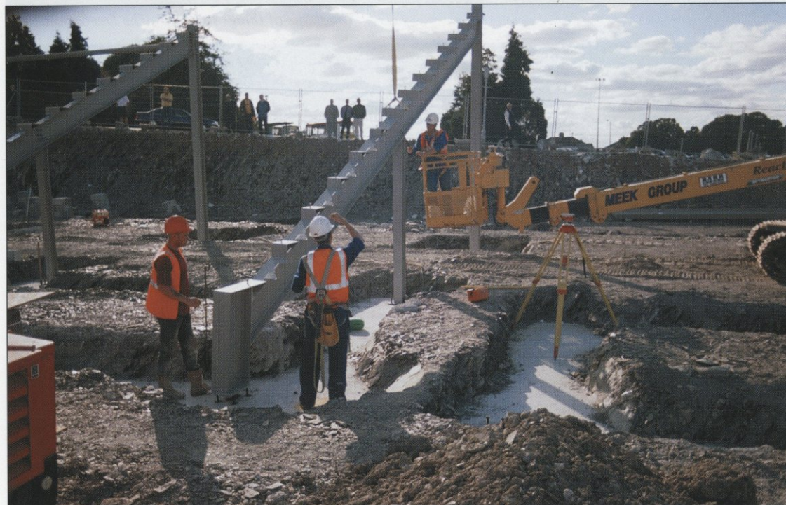
The metal work gets placed for the new Devonport Stand
