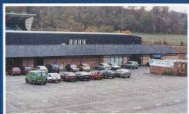
Adams Park has on site parking for over 700 vehicles.
